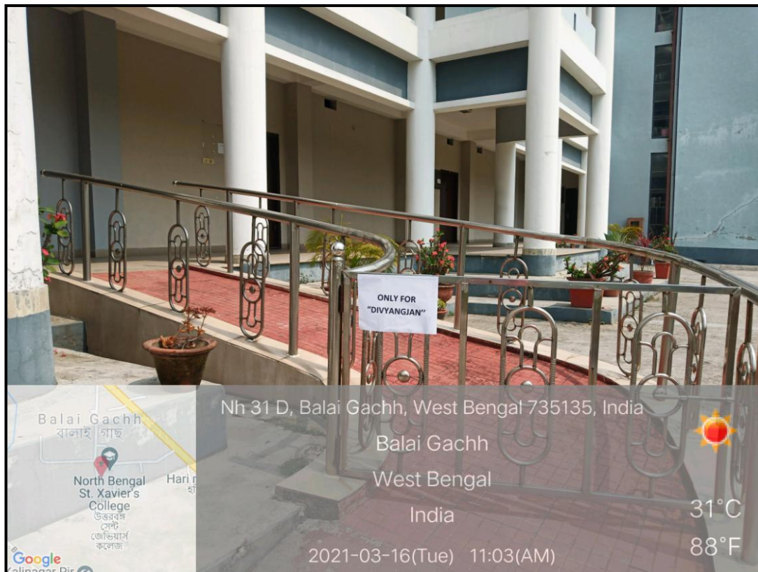
FIG. RAMP FOR DIVYANGJAN (MAIN BUILDING)
